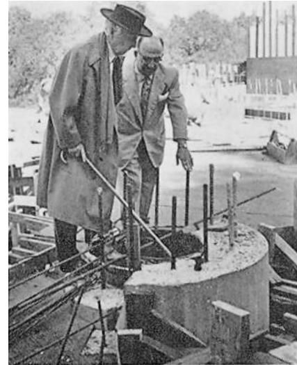
In our cover photograph Architect Frank Lloyd Wright and the author of our article are seen inspecting one of the four-foot diameter reinforced concrete columns in the Solomon R. Guggenheim Museum.
